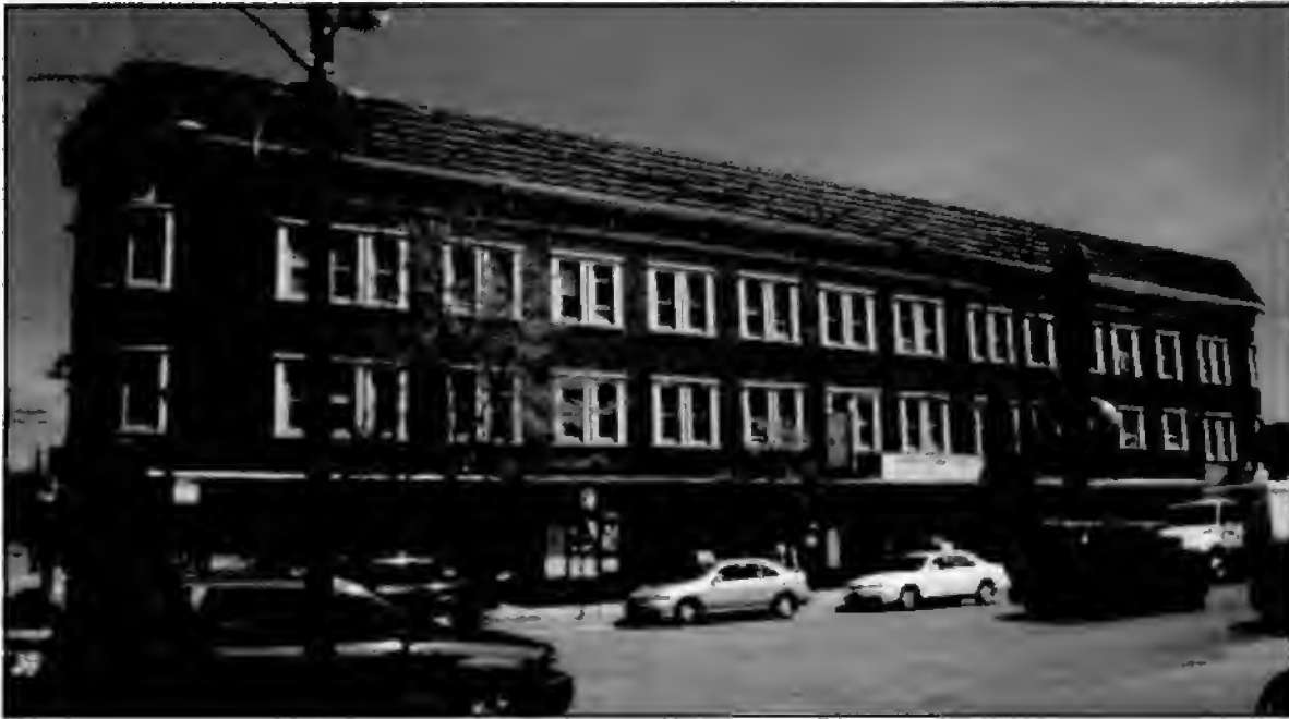
1038 –1048 West Argyle Street—the Argmore Building (1913)
